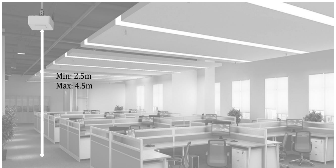
Fig-IV: Recommended Slave Gateway mounting position at height between 2.5m to 4.5m from the floor.
